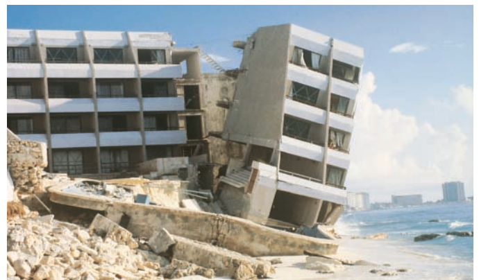
(B) Beach erosion caused by Hurricane Hugo in South Carolina made this building collapse. (Courtesy of David M. Bush/Orrin H. Pilkey, Jr.)
