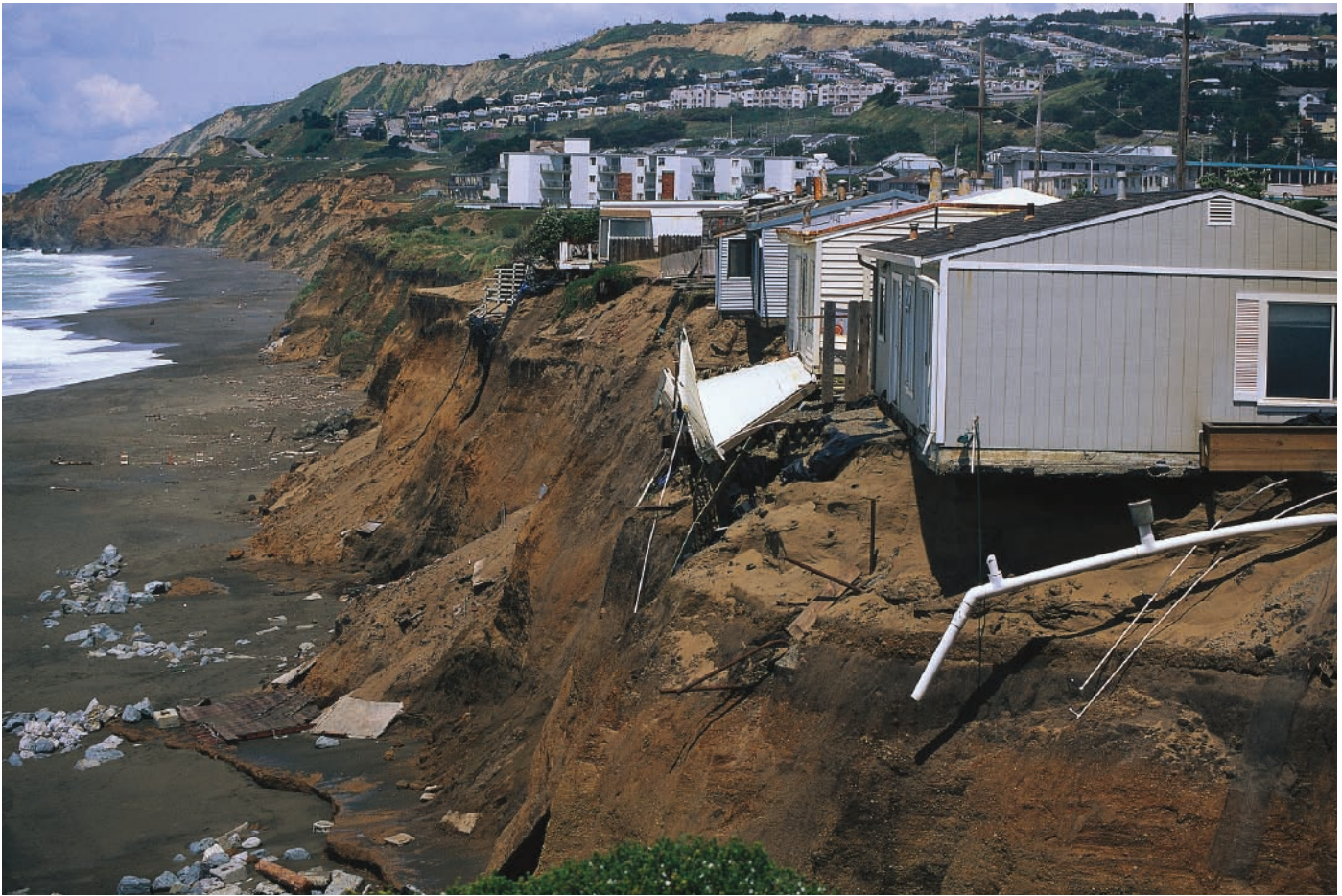
FIGURE 15.12 Erosion of sea cliffs is a major process along shorelines. This photo shows erosion of a sea cliff along the coast of California. In the last two decades, dozens of homes and hundreds of other structures have been lost or damaged because of sea cliff recession, particularly during storms triggered by El Niño oscillations. (Courtesy of CORBIS)
